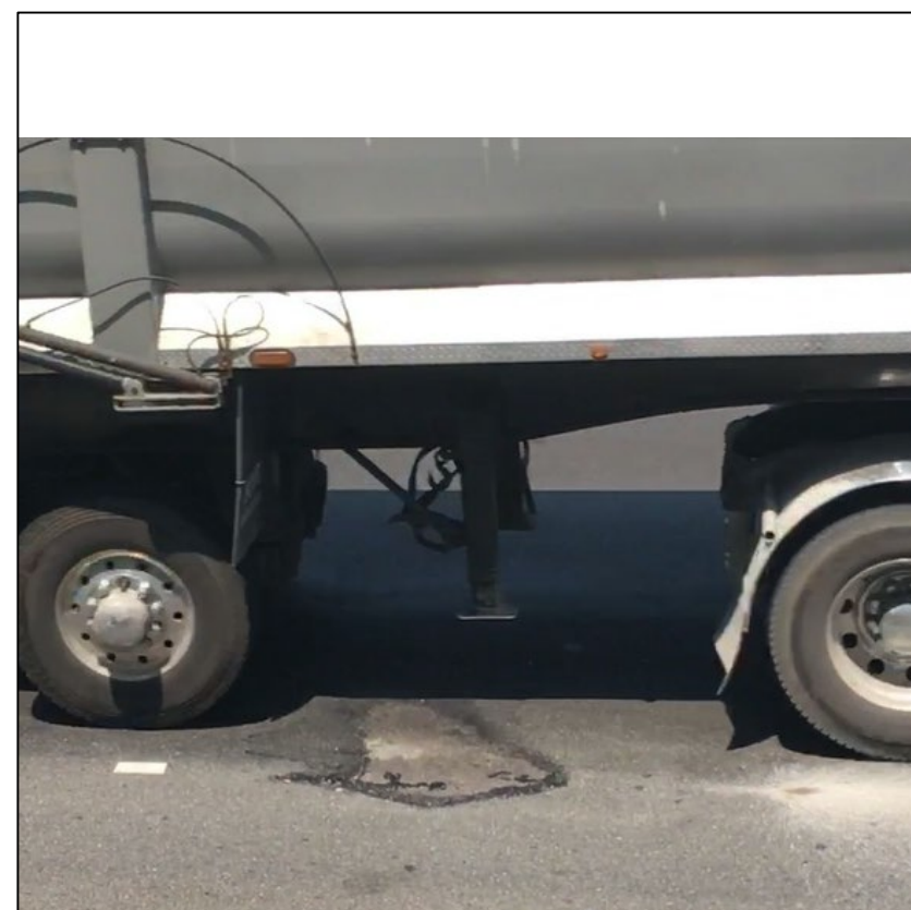
Multiple Deck Patches
