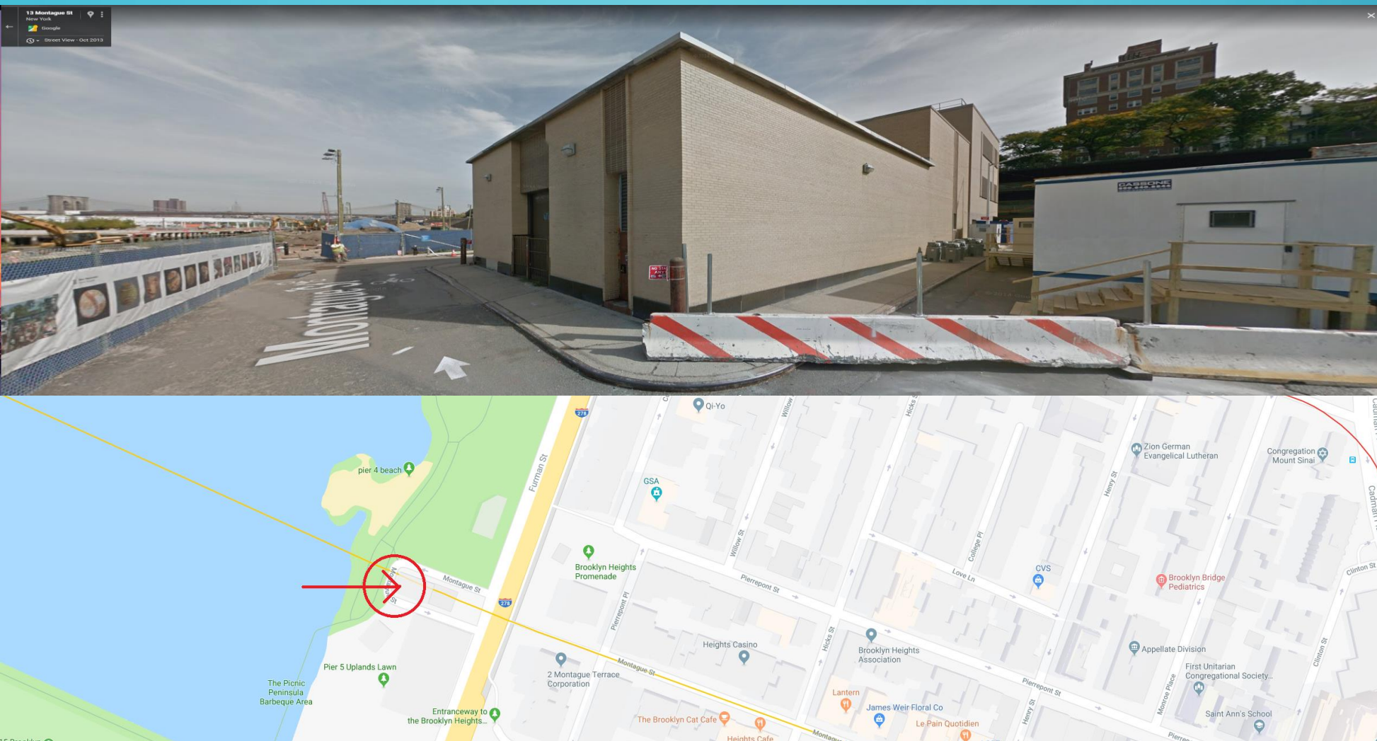
Montague-Furman Street Substation, supplies R Train
