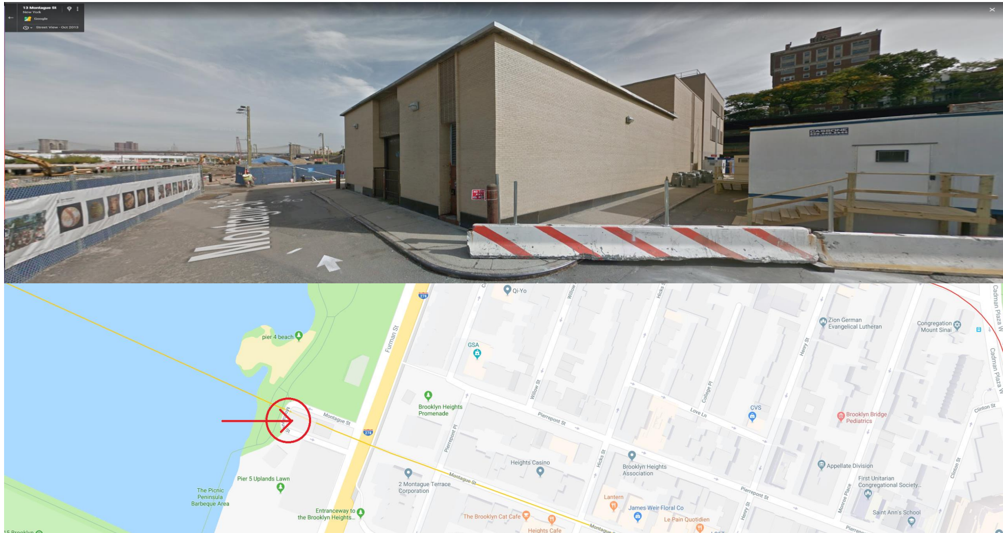
Montague-Furman Street Substation, supplies R Train
