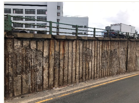
Existing condition - Hicks Street wall
