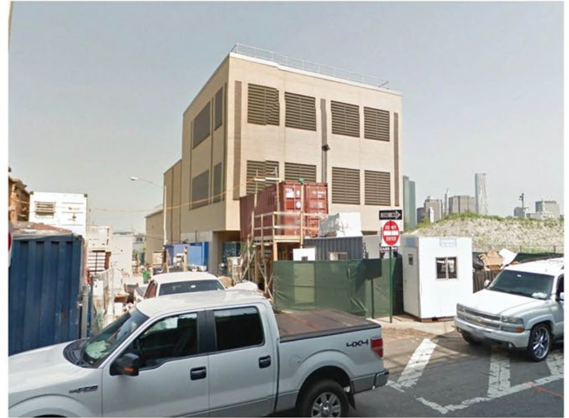
11 MONTAGUE STREET FAN PLANT
