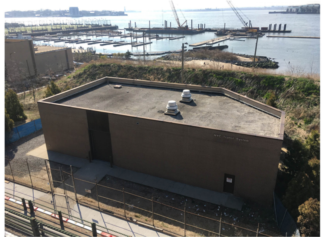
304 FURMAN STREET SUBSTATION (MTA)
