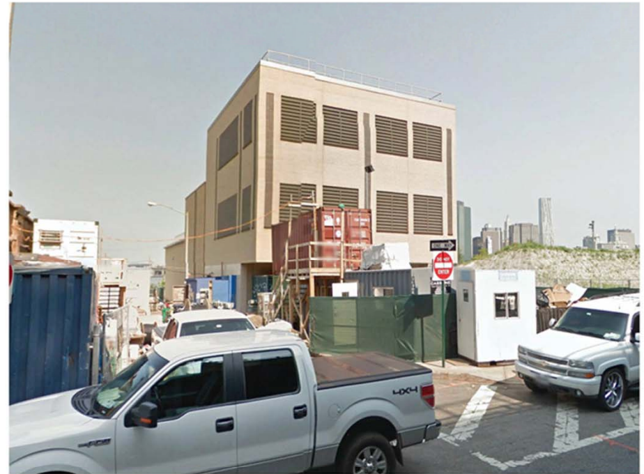
11 MONTAGUE STREET FAN PLANT
