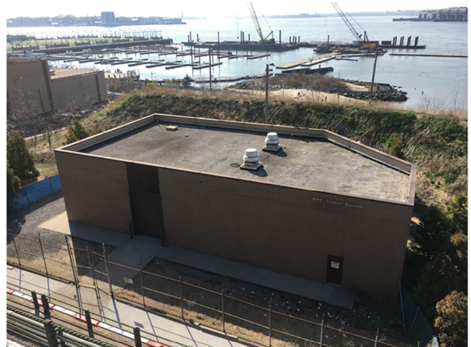
304 FURMAN STREET SUBSTATION (MTA)
