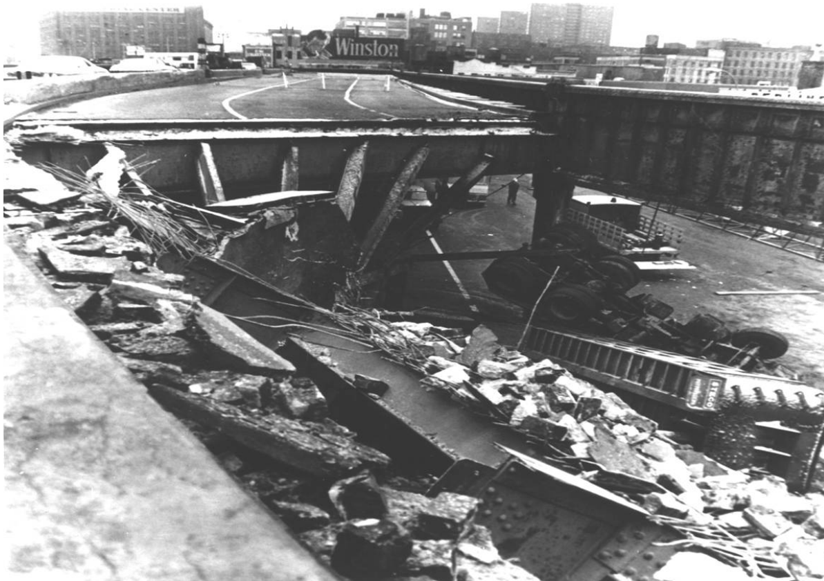
West Side Highway - 1973
