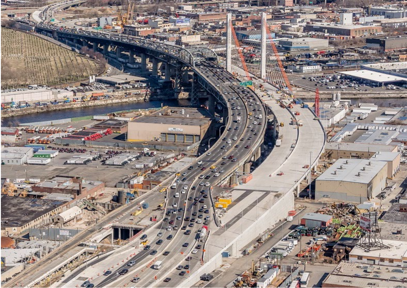
Brooklyn New Connector and Approach Alignment Next to Existing BQE March, 2017
