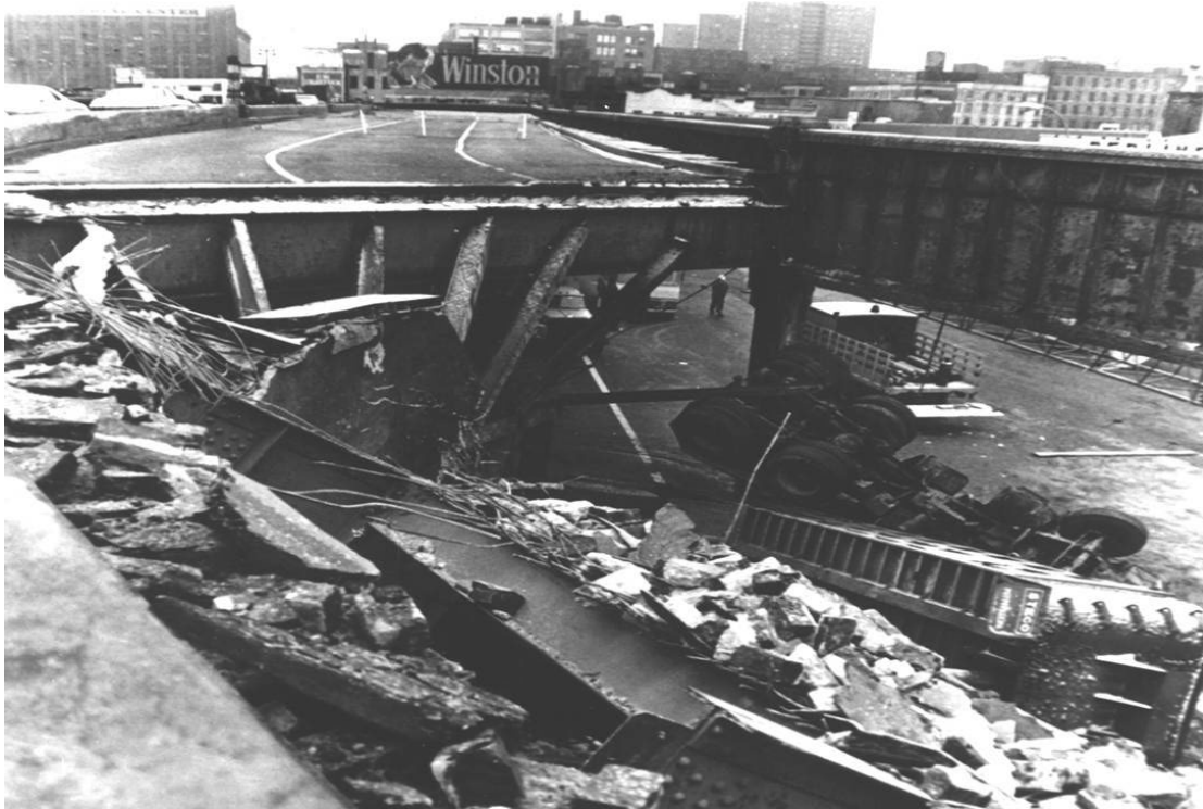
West Side Highway - 1973
