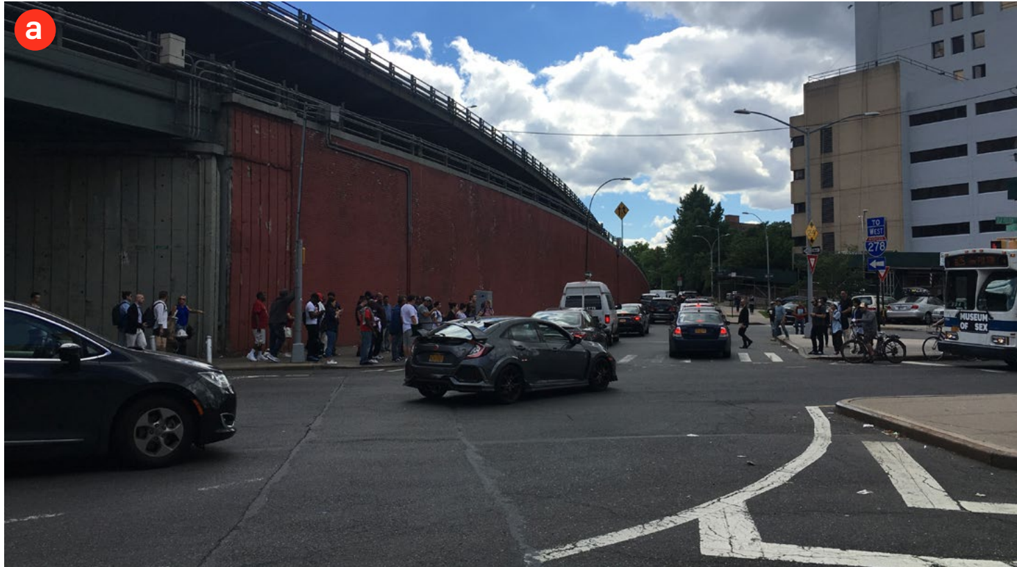
1. On-street access from Brooklyn Bridge to SI-bound BQE creating traffic congestion
