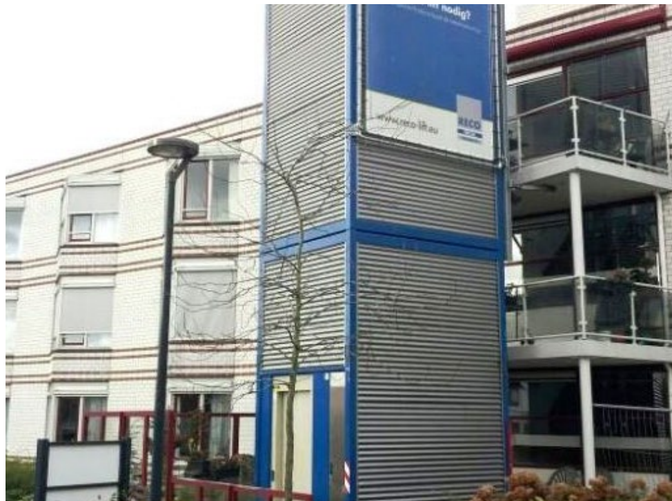
Temporary Elevator RECO Lift Solutions - UK, Netherlands, Germany
