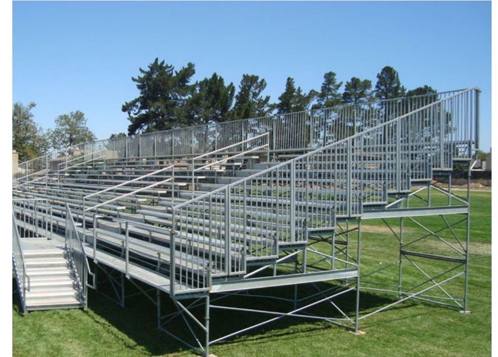
Temporary bleacher seating
