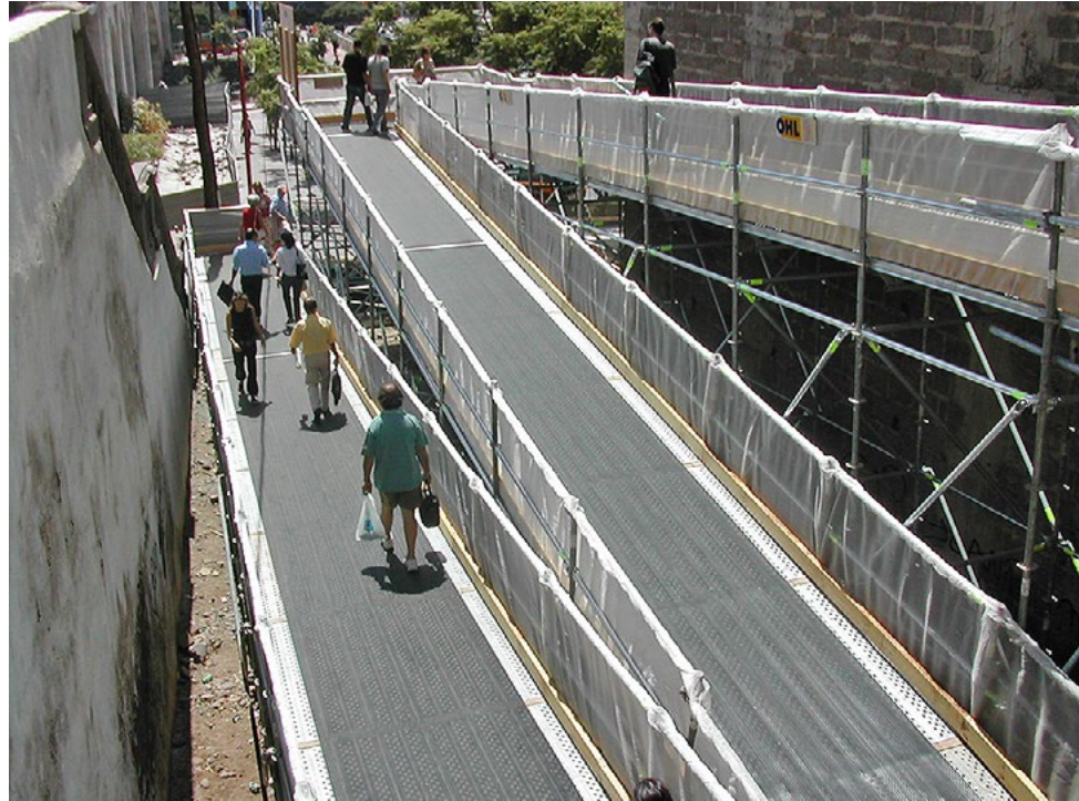
Temporary ADA ramp on scaffolding with switchbacks
