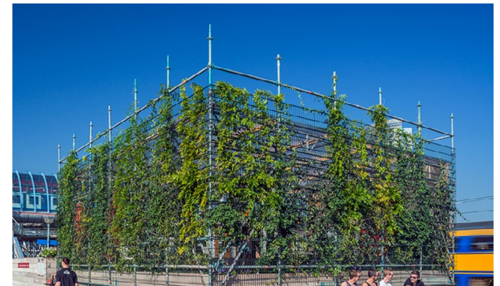
Temporary planting on scaffolding
