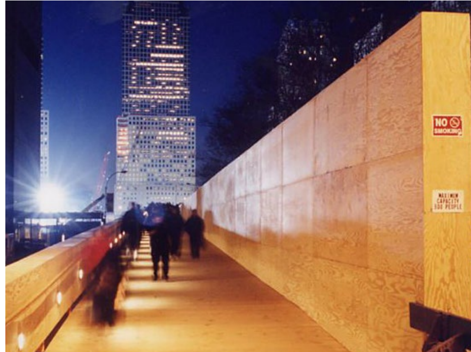
Temporary ADA ramp on scaffolding with plywood cladding
