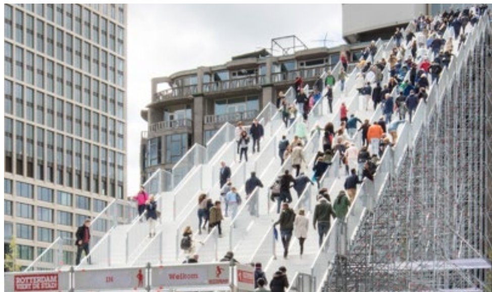
Temporary stair on scaffolding
