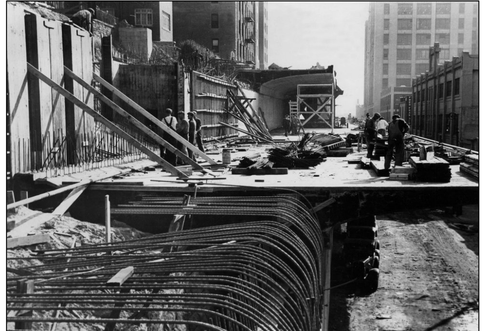
BQE under construction, 1948
