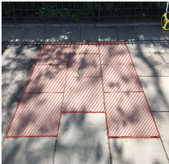
Pavers were removed for testing on the Promenade then replaced once completed
