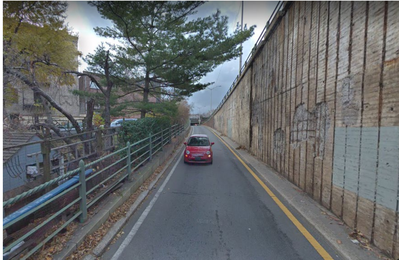
Top of BQE Ramp to Hicks Street
